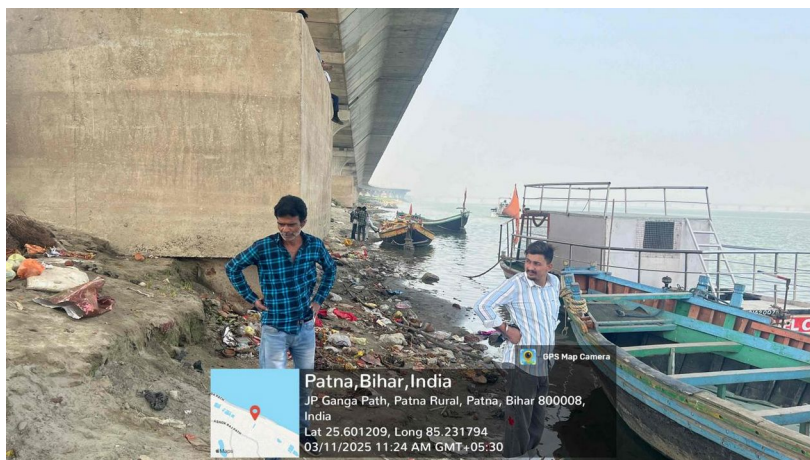
Kangan Ghat for River Front Development work at Patna City, Ganga River Patna (Jhawganj Ghat, Kangan Ghat, Kachi Talab Ghat)-200 mtr
