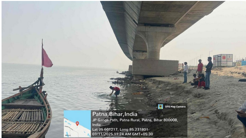
Kangan Ghat for River Front Development work at Patna City, Ganga River Patna (Jhawganj Ghat, Kangan Ghat, Kachi Talab Ghat)-200 mtr
